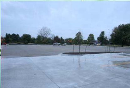
Permeable Paving: Oregon Trail Park, Olathe, Kansas
